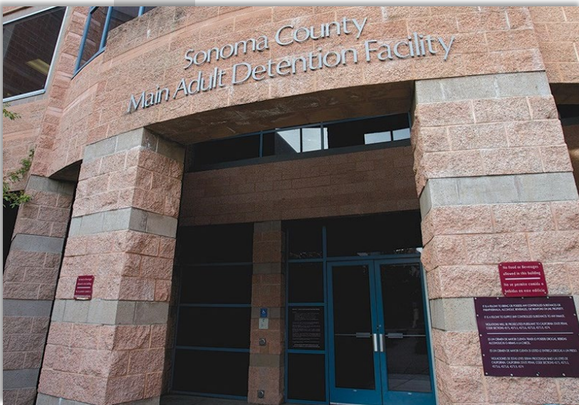
Main Adult Detention Facility
